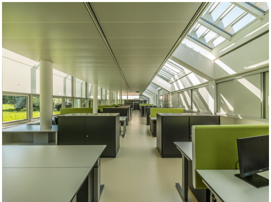
Figure 1: Interior view of the Bartenbach R&D building. The right side shows the skylights of the north side, while the left side features the fully glazed south facade with extended sunshades.
