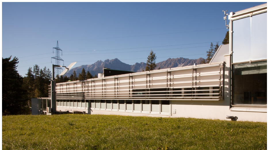
Figure 2: Exterior view of the Bartenbach R&D building showing the static daylight system on the south facade.
